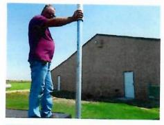
Slide the plastic sleeve over the top of the upright and down onto the tub support basket.
