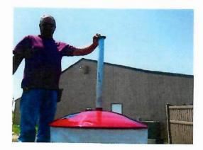
Place the collar approximately 26" to 30" from the top of the stand. If you are installing scratchers, you may even want to place it lower and then re-adjust it after you have installed the scratchers
