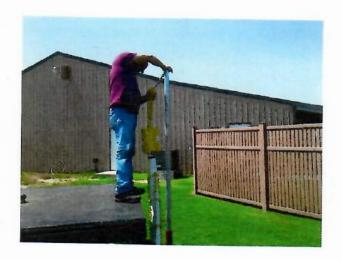
Stand on a tailgate, ladder or something safe. Hook the 3<sup>rd</sup> or 4<sup>th</sup> link in a slot at the top of the upright.
