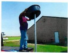
Slide the tub over the top of the upright and push it down into the tub support basket.
