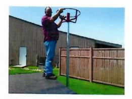
Stand on a tailgate, ladder or something safe. Using the stand you have already put together slide the tub support basket over the top of the upright and let it rest on the stand.
