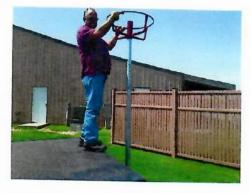
Stand on a tailgate, ladder or something safe. Using the stand you have already put together slide the tub support basket over the top of the upright and let it rest on the stand.
